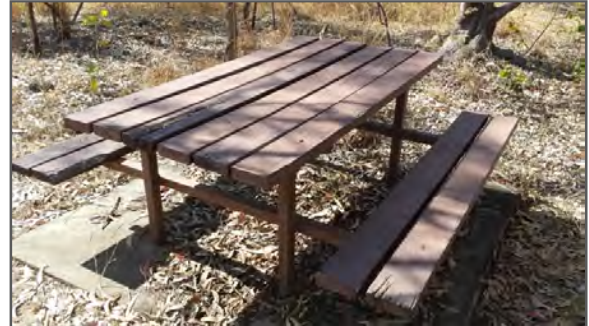
Facilities in some areas of the Reserve are tired and need replacing
