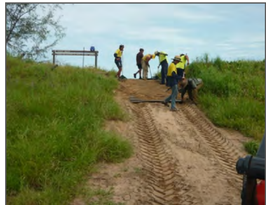
Larrakia Rangers constructing new beach access boardwalks in the Reserve
