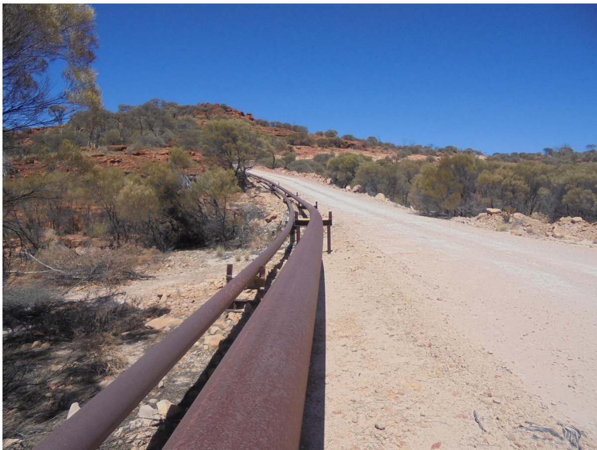
Figure 6-5 Typical flowline and associated pipe stands at PVGF
