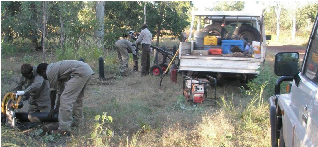
Park Rangers and flexible employment staff install bollards at Djarrung campground.
