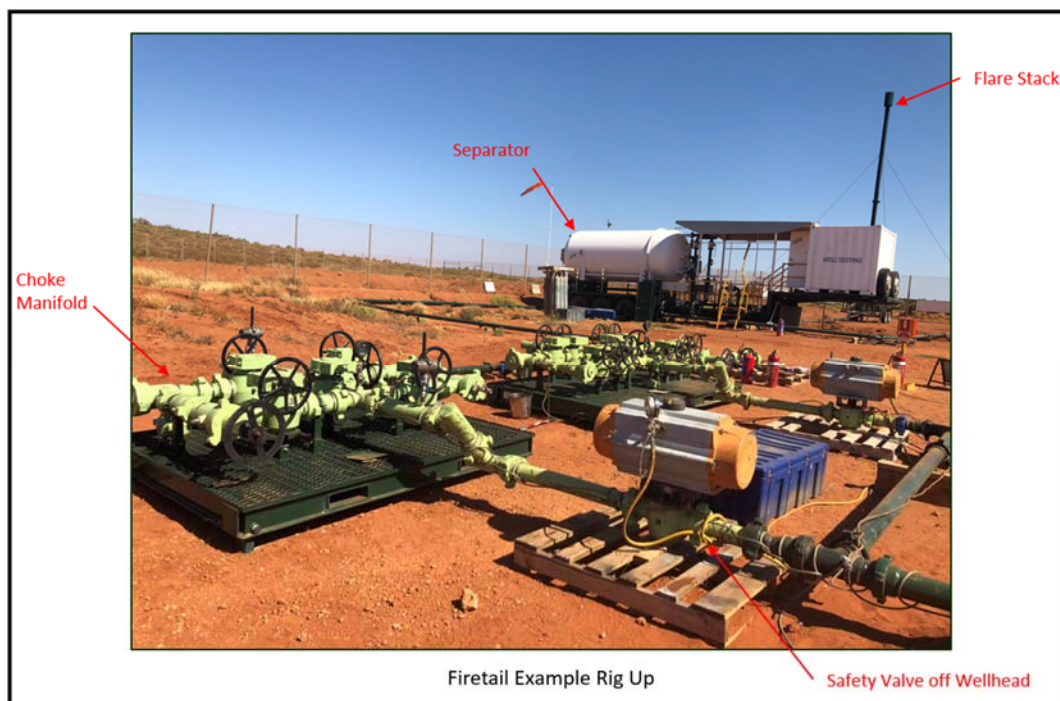
Figure 3-24 Example Well testing Flare Set Up.
