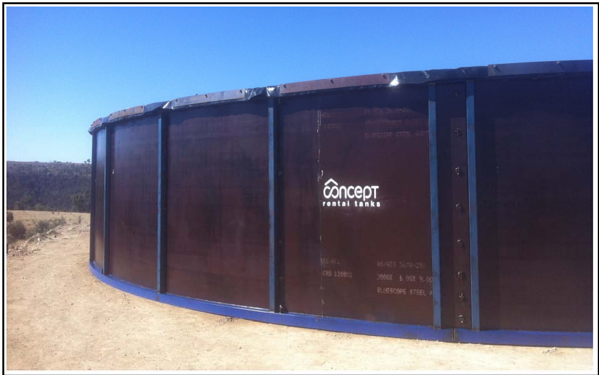
Figure 3-19 Above ground storage tank
