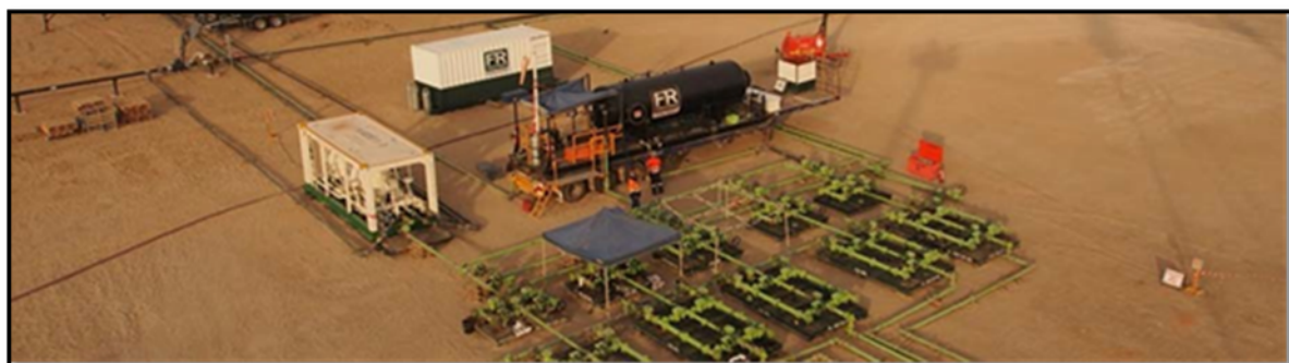
Figure 3-26 – Photo of Separator Package Installed on Multiple Well Pad in Cooper Basin
