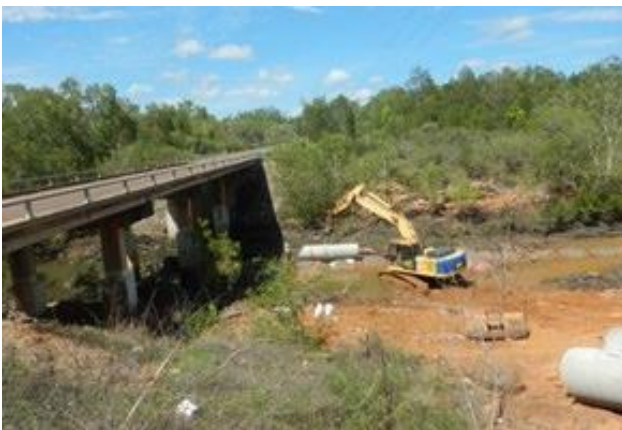
Plate 10: Bund wall construction at Cox Peninsula Bridge
