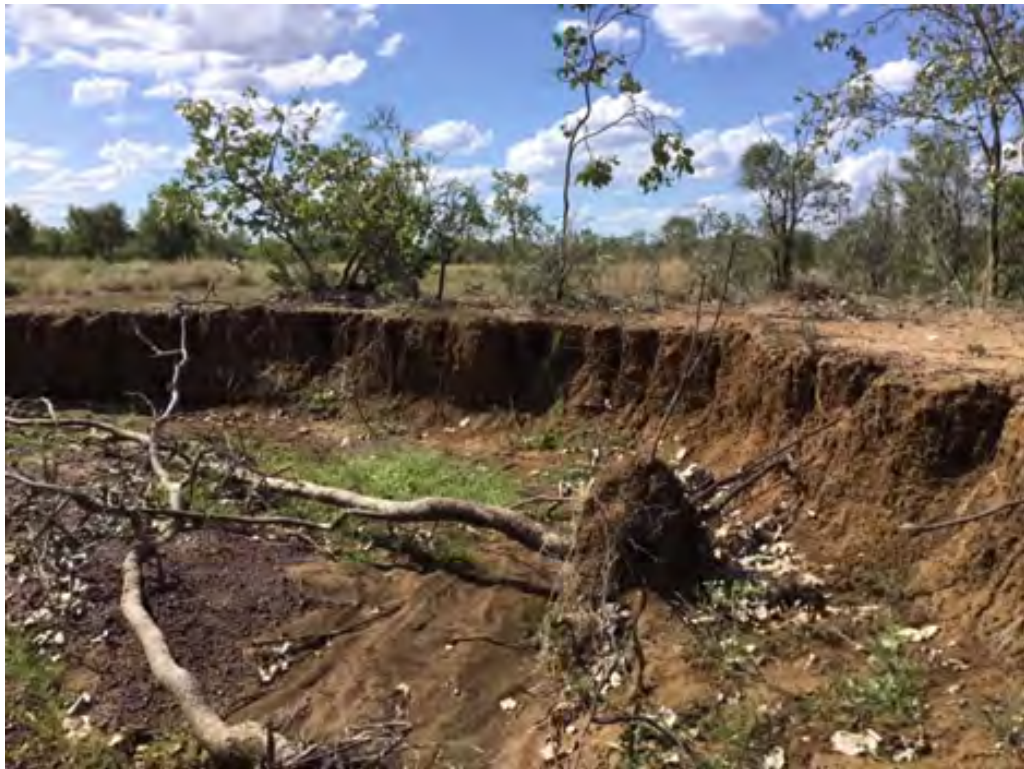
Plate 6. Actively migrating creek channel, exhibiting erosion causing tree fall and a steep outer channel margin exposing depth of loose clayey sand sediment. Located in the Tanumbirini North Area. Aboriginal stone artefacts are absent in the section along the channel bank or within the channel.
