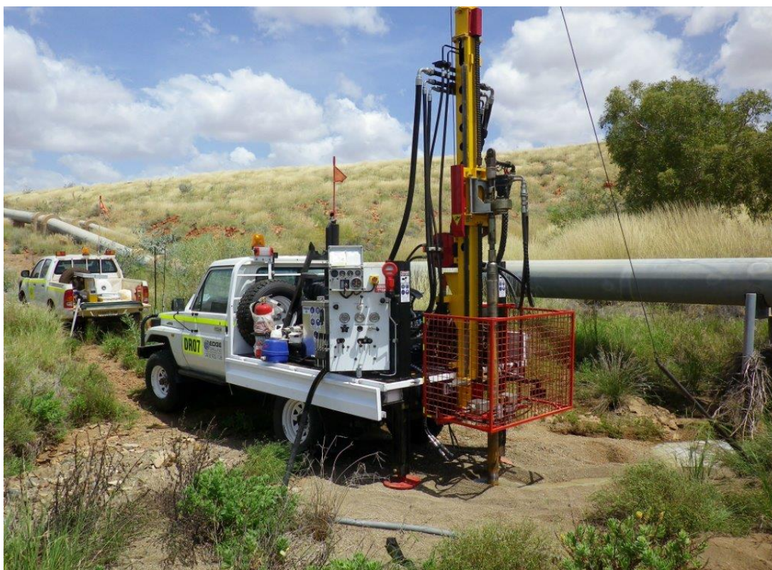
Figure: Truck mounted rig preparing shallow hole to install tiltmeter.
