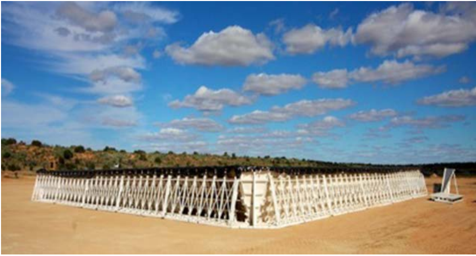
Figure: Above ground storage ponds used for frac make up water storage and frac flowback water storage in the Cooper Basin, (Santos 2013)
