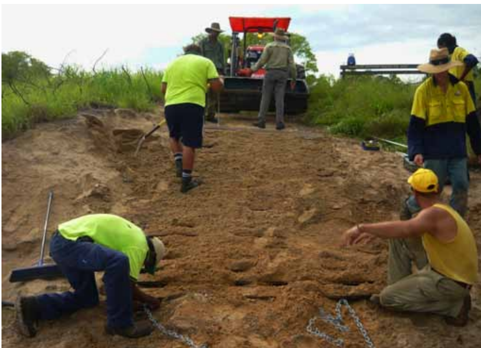
In 2012, Larrakia Nation Rangers fabricated and installed 166 m of boardwalk for 6 Casuarina Coastal Reserve beach accesses. Concrete sand anchors also had to be fabricated and installed. Pictured here are Larrakia Nation rangers connecting the boardwalks to the sand anchors prior to stretching and final dressing. The installation was done in collaboration with the Darwin PWC rangers.
