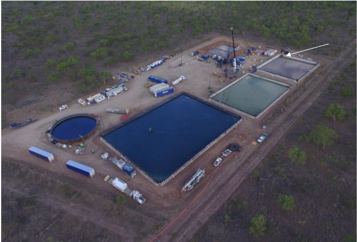
Figure 22: Amungee NW-1 Well Testing image. Note, three of the 4 tanks will be enclosed with a working evaporation tank.
