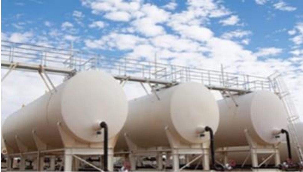
Figure 21 Example of condensate storage tanks (image provided for indicative purposes only)
