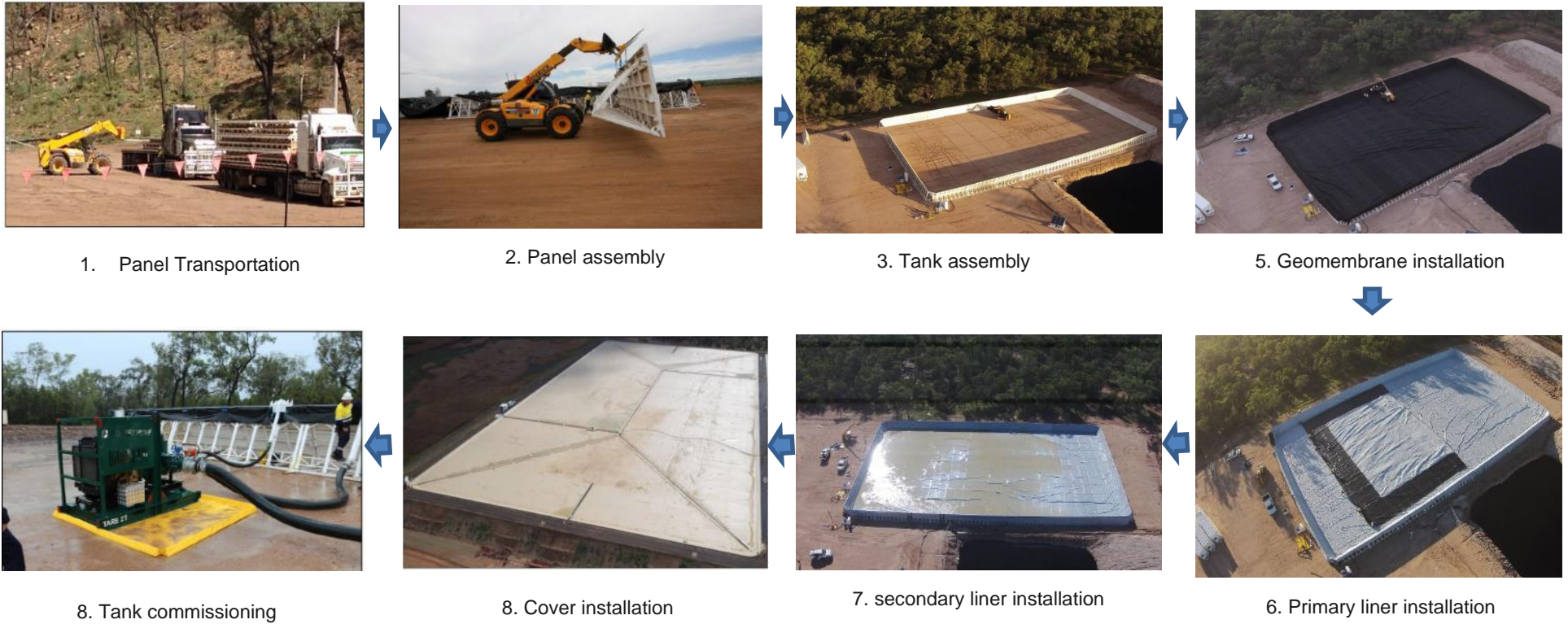
Figure 13 Wastewater tank construction process
