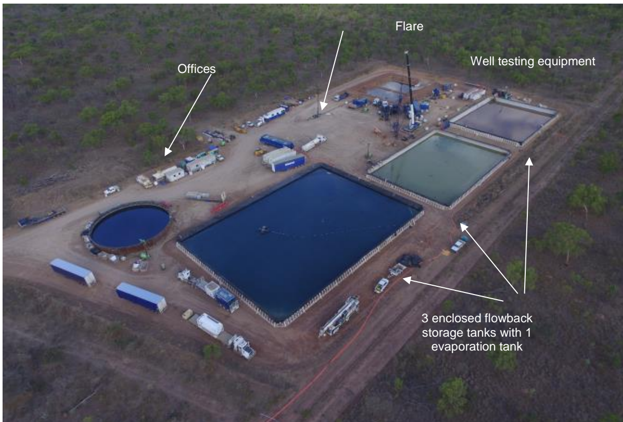
Figure 17: Amungee NW-1 Well Testing image. Note, three of the 4 tanks will be enclosed with a working evaporation tank.
