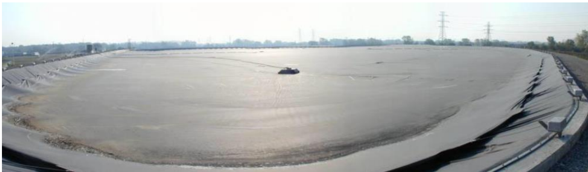
Figure 24: Covered water storage example.
