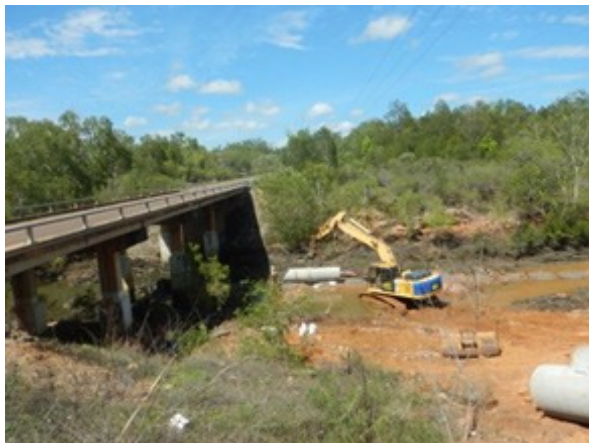
Plate 9: Bund wall construction at Cox Peninsula Bridge
