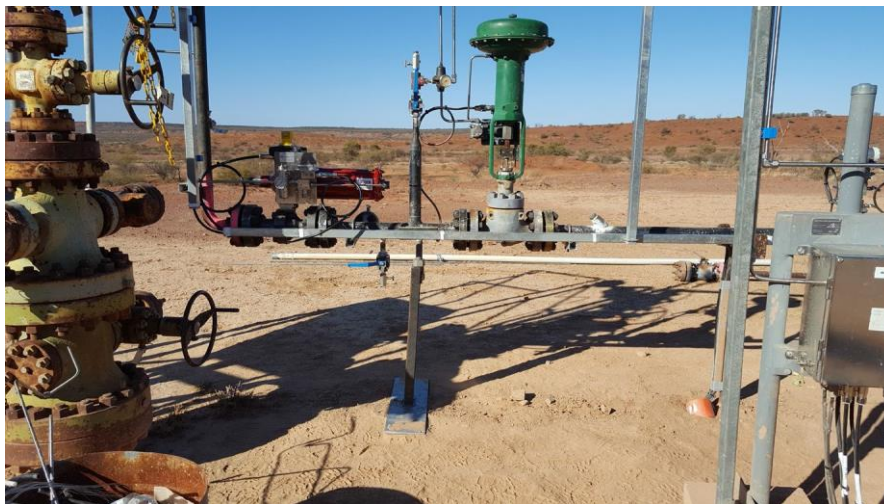
Figure 4-6 Example of typical metering instrument, skid
