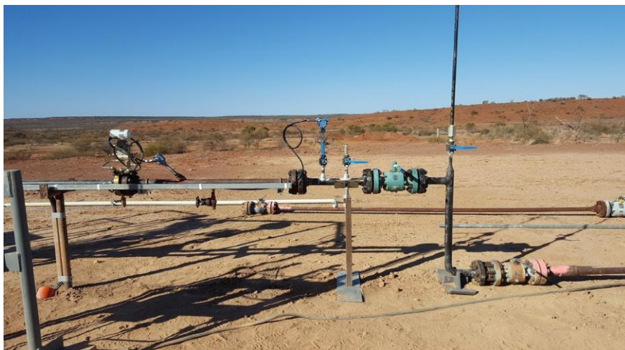
Figure 4-7 Example of typical control valves
