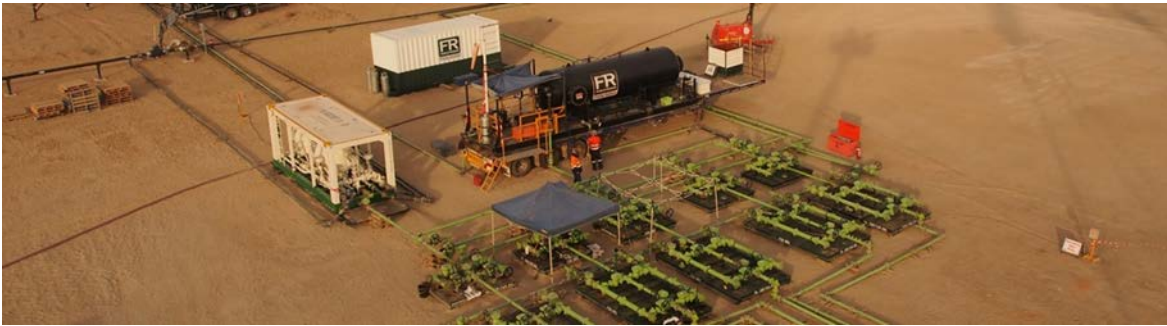
Figure 3.20: Flow testing separator rig up on a pad location. (Farley Riggs 2014)
