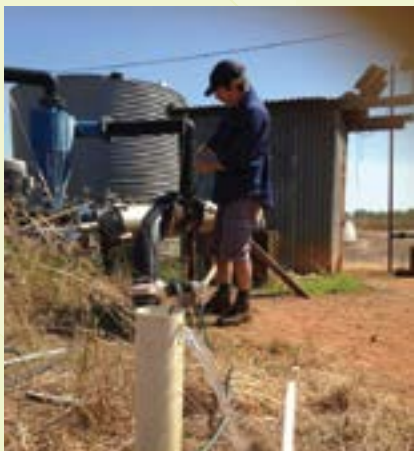
Photo: Measuring bore standing water level - Rodney Metcalfe, Water Resources Division.
