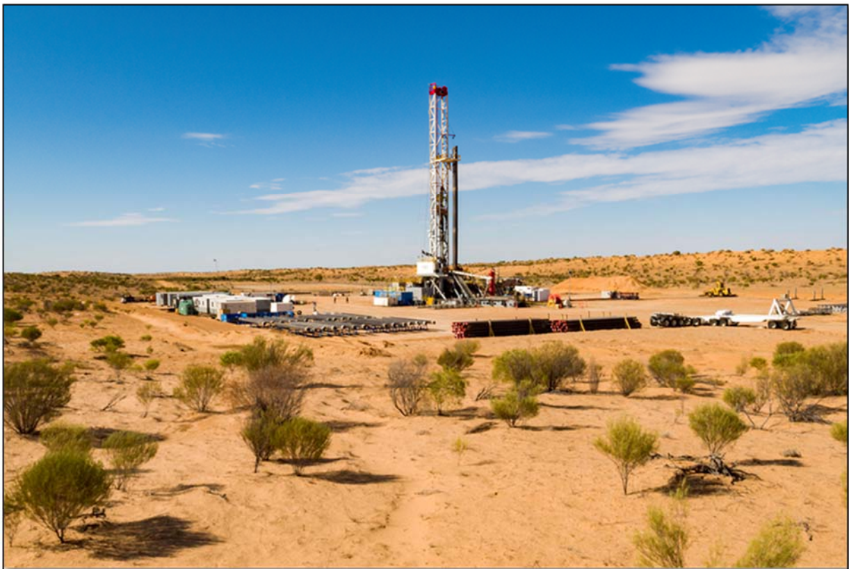
Figure 3-4: Ensign Australia Ltd ADR 1500 drilling rig
