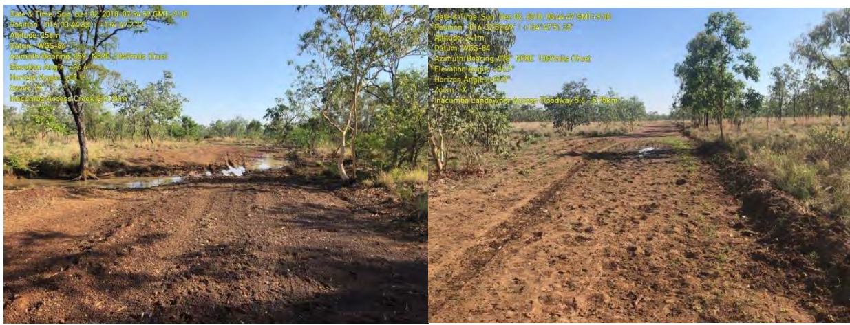
Chainage 5.4 drainage line crossing (left) and chainage 5.6-5.7 floodway area (right)
