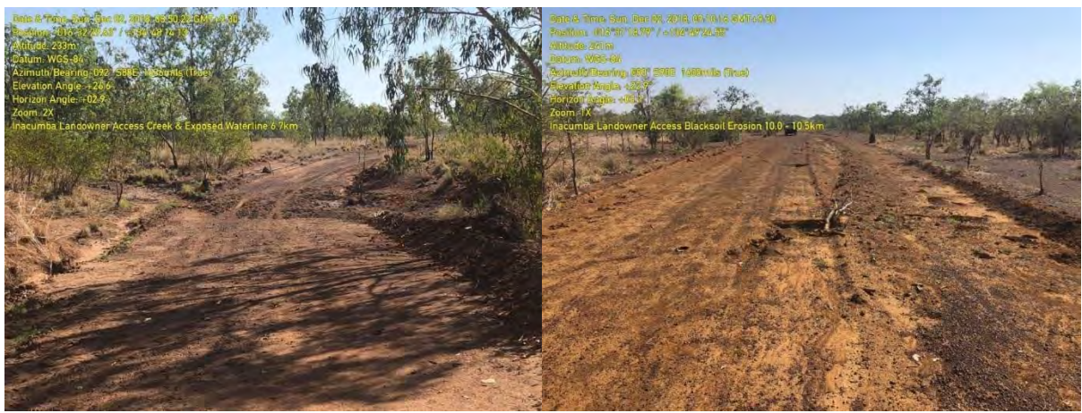
Chainage 6.7 drainage line crossing and chainage 10.5 drainage line crossing
